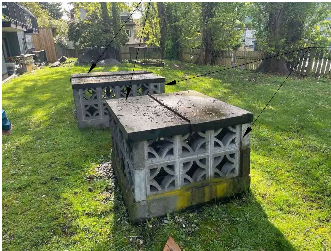
1 VENTS OVER PARKADE AT SOUTH SIDE OF THE BUILDING SCALE: N.T.S.
