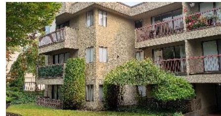
Figure 1 - Overview of building
