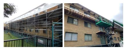
12.2 Balcony soffits were observed to be excessively fastened, leading to irreversible damages at the removal. All soffits were to be replaced with new. Approximately 455 sqm was confirmed.
