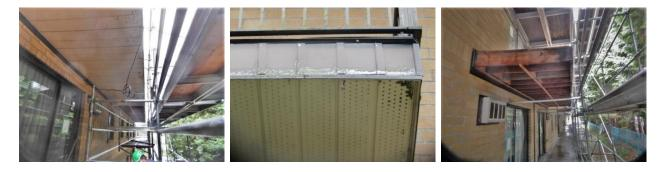
12.3 Concrete delamination was found in various areas on the second floor decks. Approximately 29 sqm more was confirmed that is needed to be repaired to complete the work.
