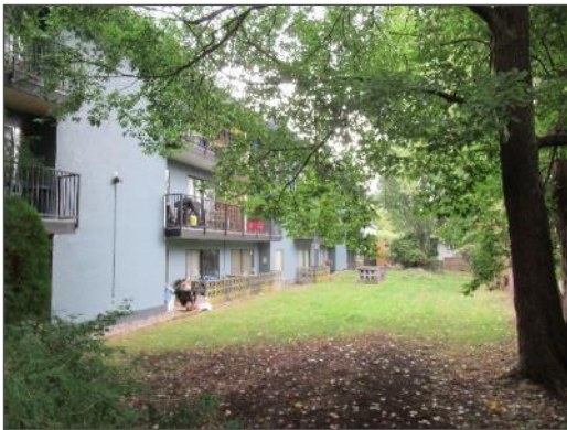
View of the soft landscaping on the south portion of the Site.
