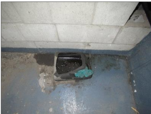
View of the “oil collection system” used in the site as well as minor oil stains on the floor.
