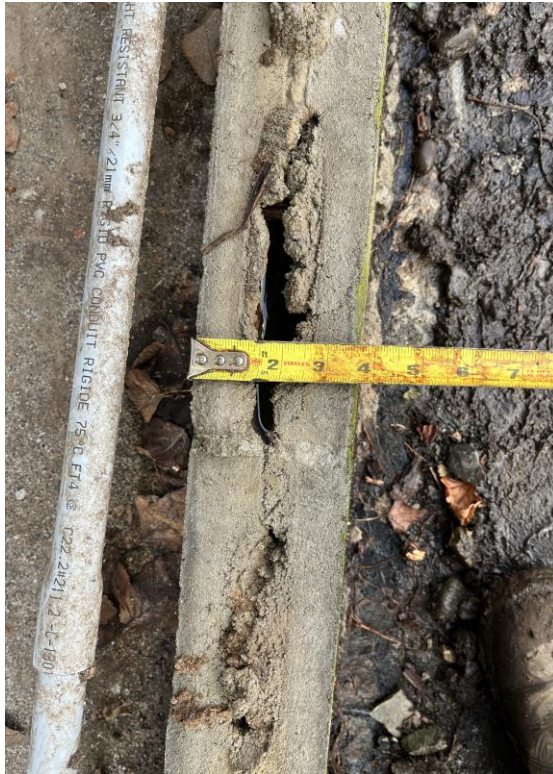
Balcony Concrete Curb 1
