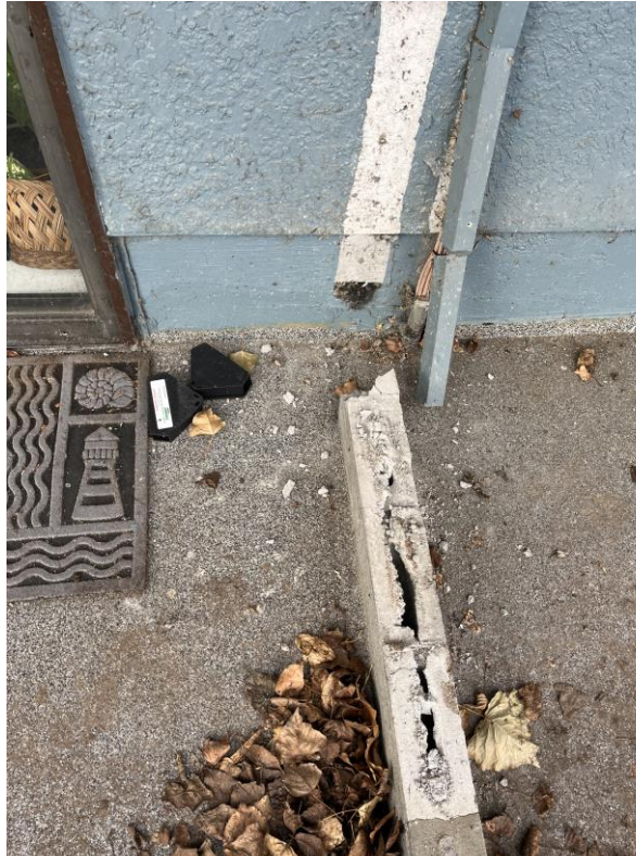
Balcony Concrete Curb 3
