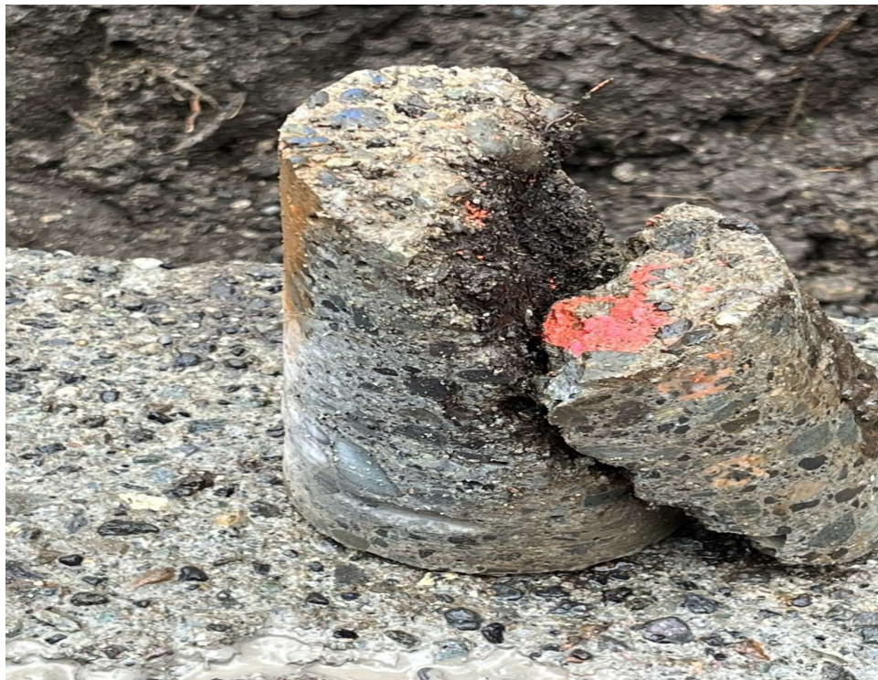
Picture 3: Cored cylinder from concrete slab
