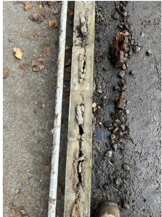
Balcony Concrete Curb 2
