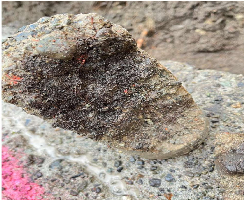
Picture 4: Cored cylinder from concrete slab
